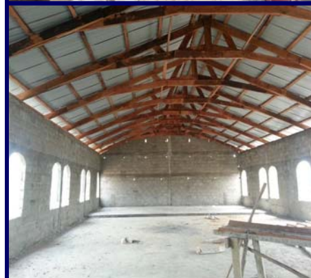
Inside view of St. Paul construction towards the altar area.
