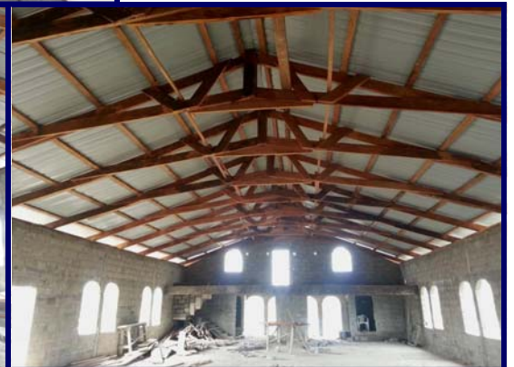
Inside view of St. Paul construction from the front entrance.
